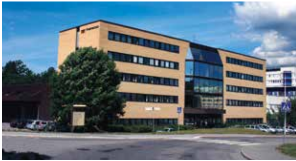
Terco headoffice and factory outside Stockholm, Sweden
